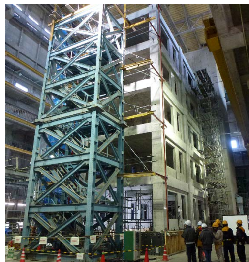
Full scale specimen at South area
