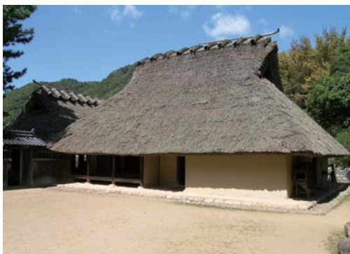
Hakogike house in Kobe, Hyogo Prefecture
