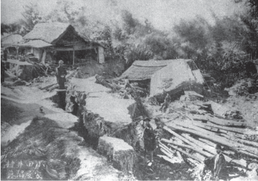
Damage to wooden buildings in the Nobi earthquake of 1891, centered on Gifu and Aichi prefectures
