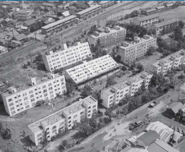
Photo 1: The Niigata Earthquake of June 16, 1964, caused the four-story buildings of Kawagishi-cho Apartments to list significantly off center or topple altogether.
