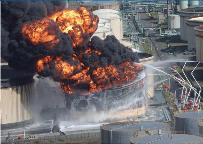
Photo 2: An earthquake off the Pacific Coast of Hokkaido in 2003 caused oil storage tanks to catch fire at a refinery in Tomakomai, over 200 km from the epicenter, when the naphtha and petroleum in the tanks shook in synchronization with the slow moving tremors.
