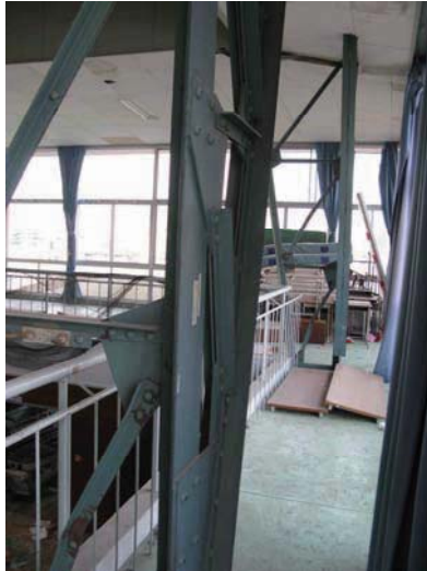
(a) Latticed column
