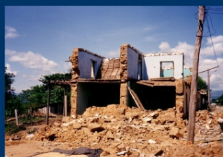
Damage to Tapial construction (1990 Peru EQ)
