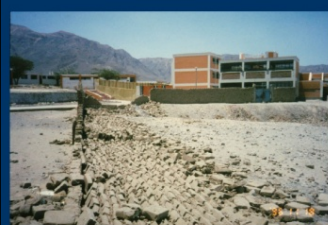
Damage to Adobe (sundried mud block) construction (1996 Nazca, Peru EQ)
