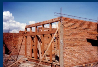
Wood frame for door sash can support brick wall.
