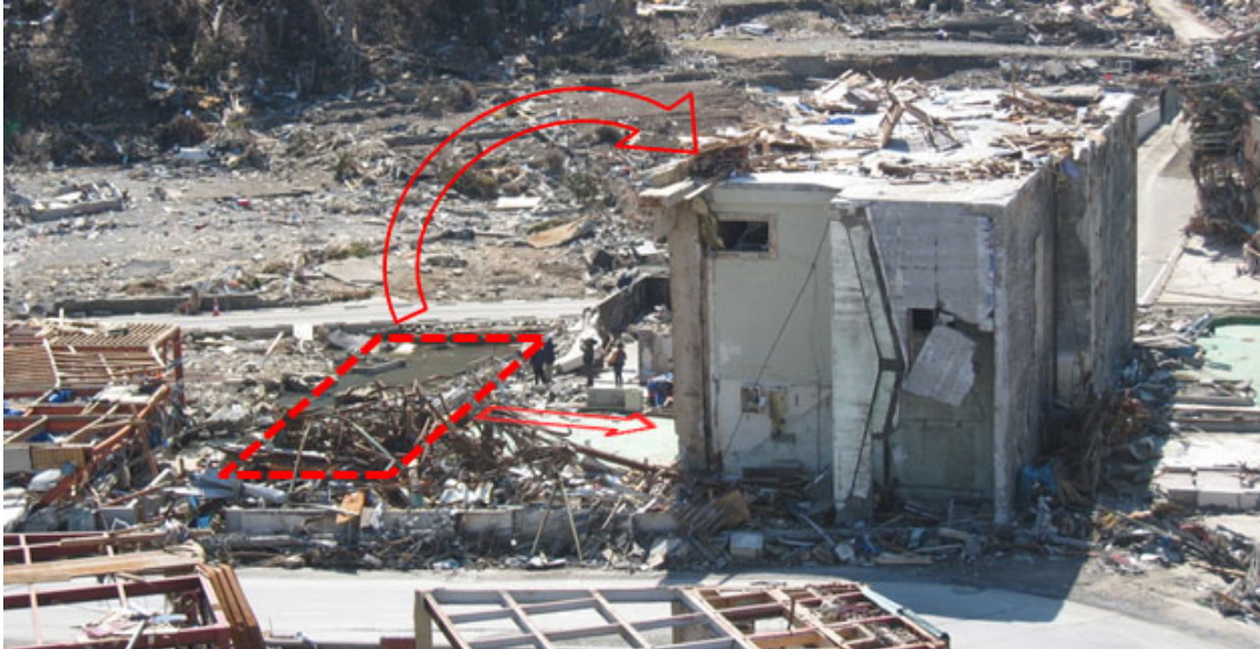
Figure 8 Overturning of a reinforced concrete warehouse in Onagawa city
