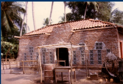
Un-reinforced brick masonry with no columns and beams (Java, Indonesia)
