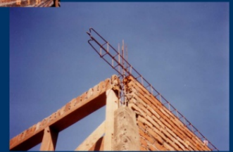
Damage to Tapial construction (1990 Peru EQ)
