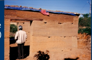
Tapial is cast-in-place mud (rammed earth) construction (1990 Peru EQ)
