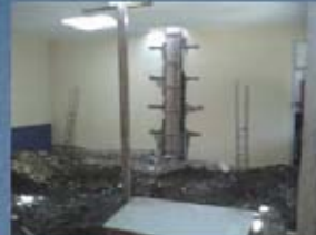
Retrofitting work (Krishna Pribadi)
