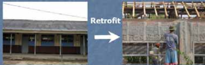
Retrofitting project of SD Padasuka II, Indonesia
