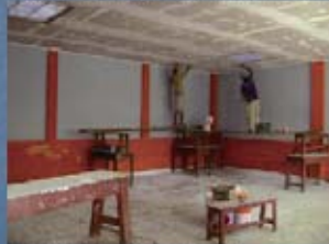
Finishing work (Krishna Pribadi)
