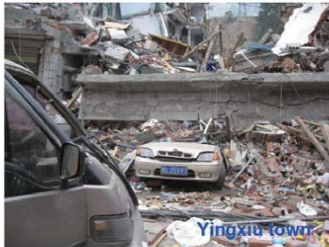
The building collapsed and the cars crushed
