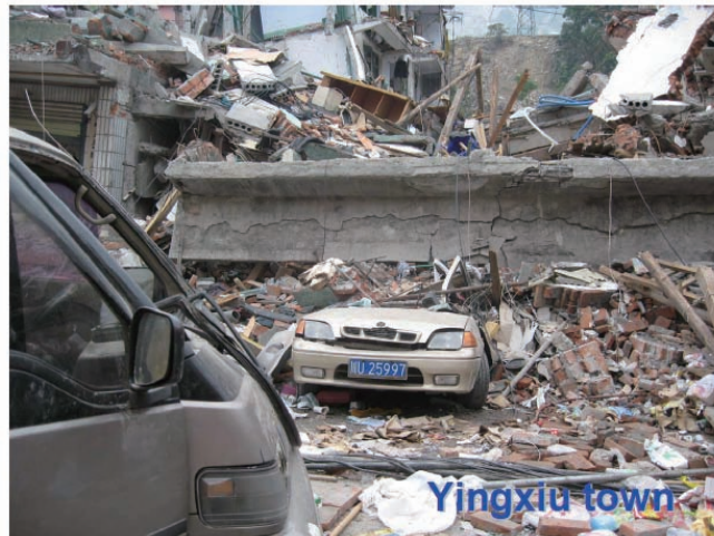
The building collapsed and the cars crushed
