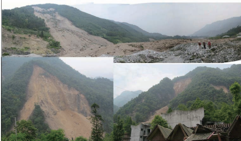
Earth slide and collapse caused by the earthquake
