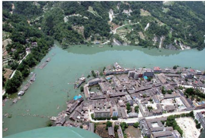
Tangjiashan barrier lake caused by Wenchuan
