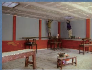
Finishing work (Krishna Pribadi)
