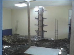
Retrofitting work (Krishna Pribadi)
